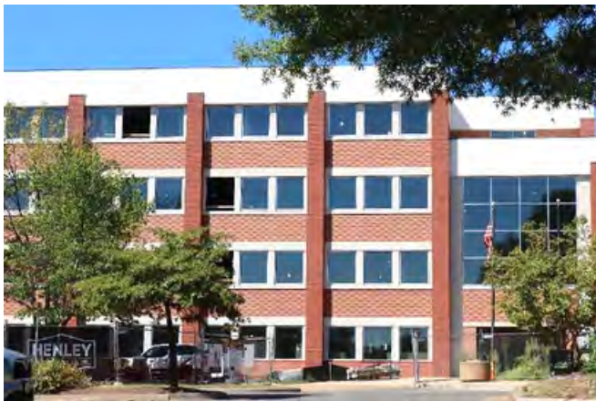
The renovations to City Hall are ongoing.
