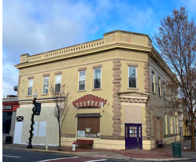
Two new restaurants on Center Street to include Gadfly Gastro Pub (9110) and Zengo (9112) are currently under construction.
